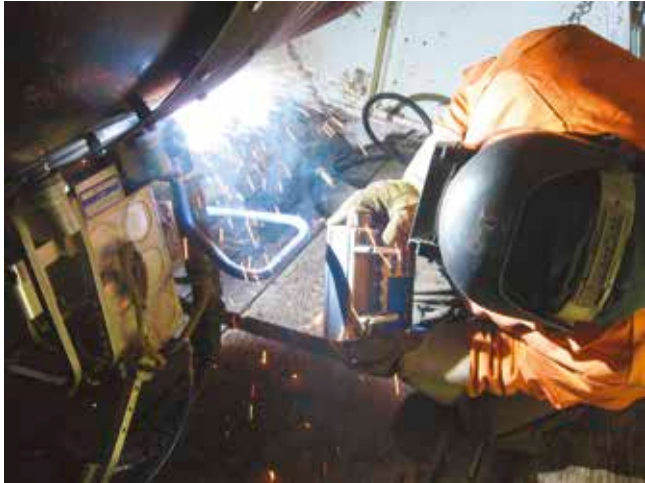
Figure 8. Mechanised welding operator welding vertical-up, at the bottom of the pipe.
