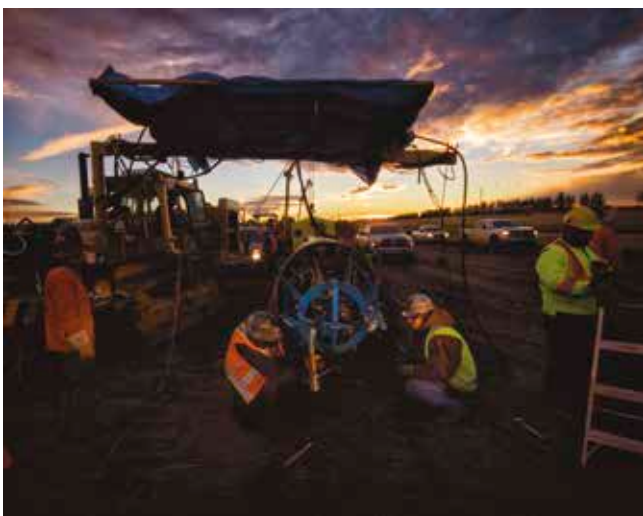
Figure 3. Crew inspecting the internal line-up clamp.
