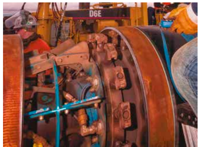
Figure 4. Pipe incoming to the internal line-up clamp.
