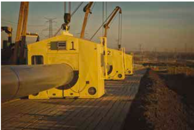
Figure 2. Mechanised welding 'shacks' on rig mats.
