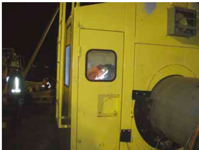
Figure 7. Mechanised welding operator welding inside a 'shack'.
