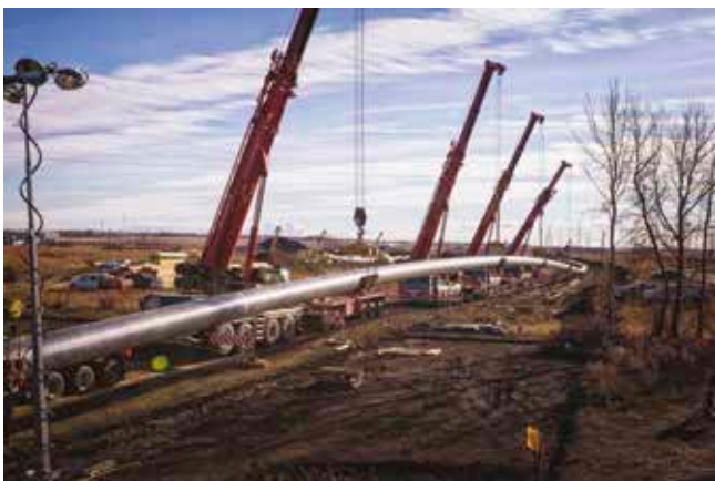
Figure 10. A pipeline section being lowered-in.
