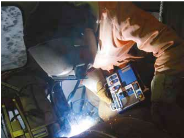
Figure 9. Mechanised welding operator welding vertical-up, at the side of the pipe.
